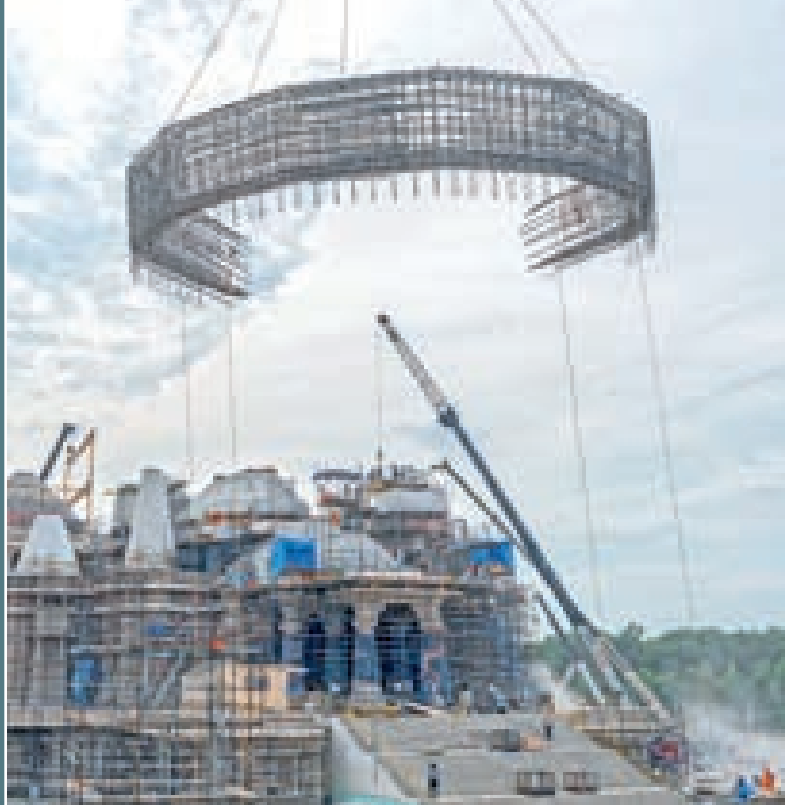
Frame of iron rods (rebars) lifted for on-site construction
