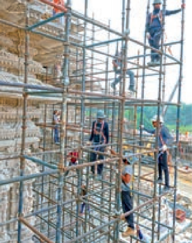
Erecting a scaffold on-site
