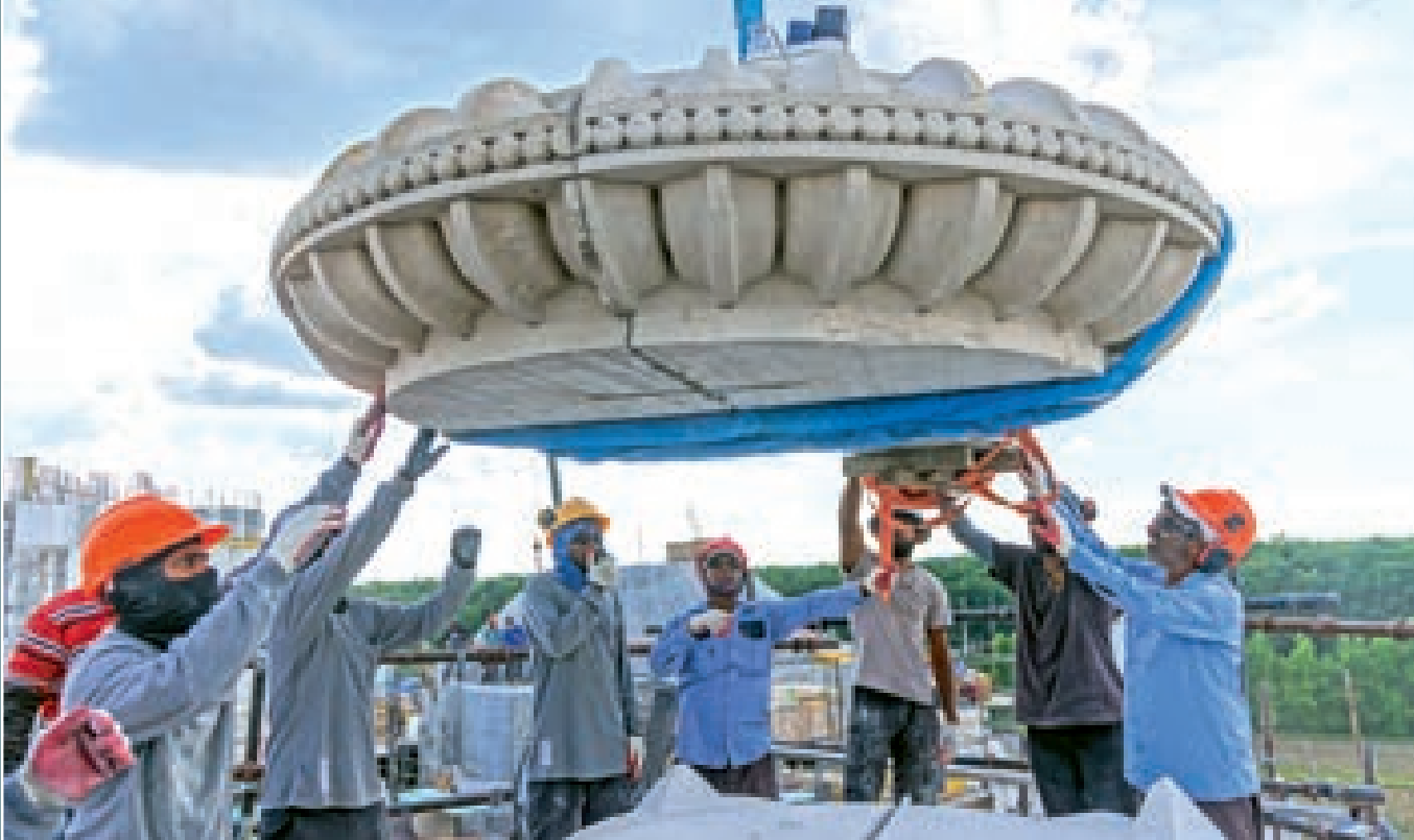
Placing an amalaka on one of the shikhars
