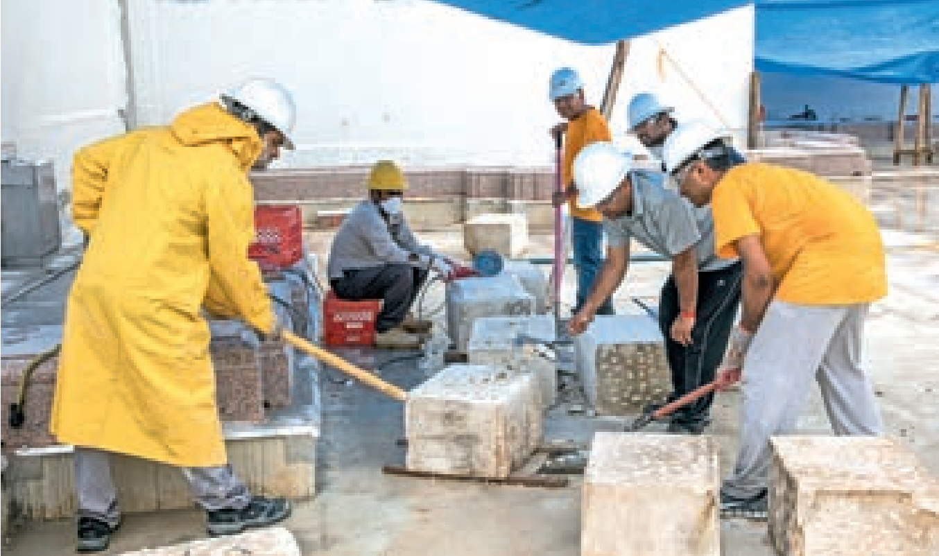
Moving a stone for placement
