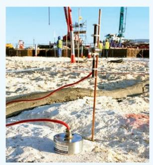
A sensor placed in position upon the sandstone in the mandir foundation
