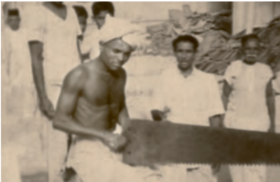
Cutting stones with a saw
